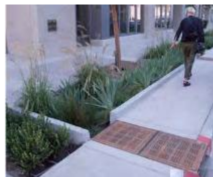
In addition, they can be designed to filter stormwater run-off from street, per BOE Green Street standards; if there is a raised curb around the parkway and curbside parking as in this example, the curb access strip must be wider than 2 feet
