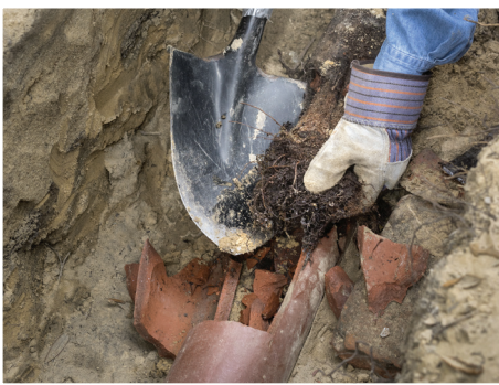
Plumber making repairs on private lateral
